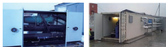
Fig.5,6 - Stationary and modular arrangement of heat pumps
